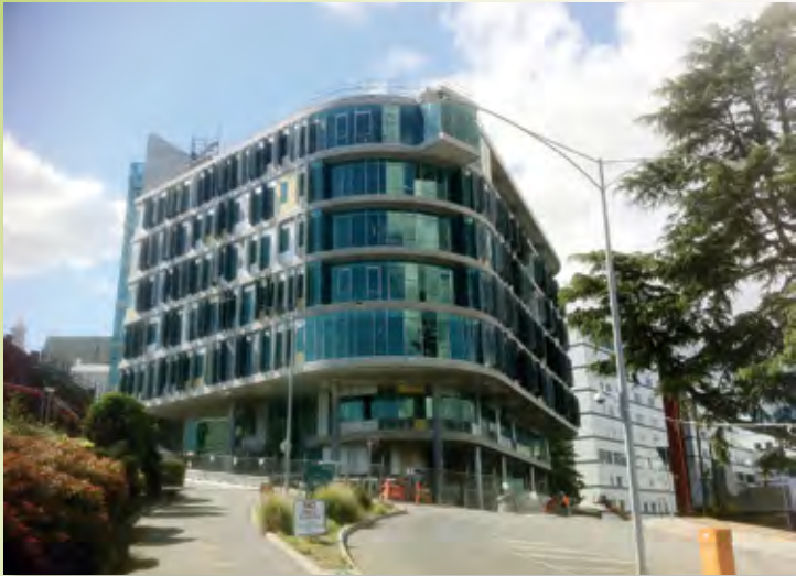
External structure almost finished
