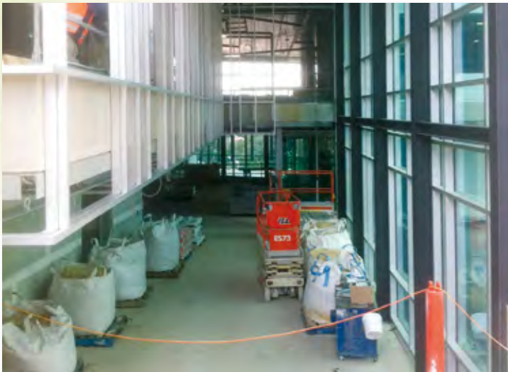
Full steam ahead on internal fitout
