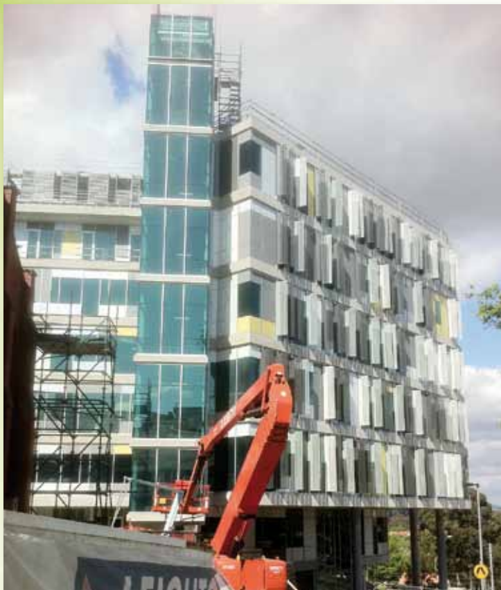
View of rear stairwell - facade nearing completion
