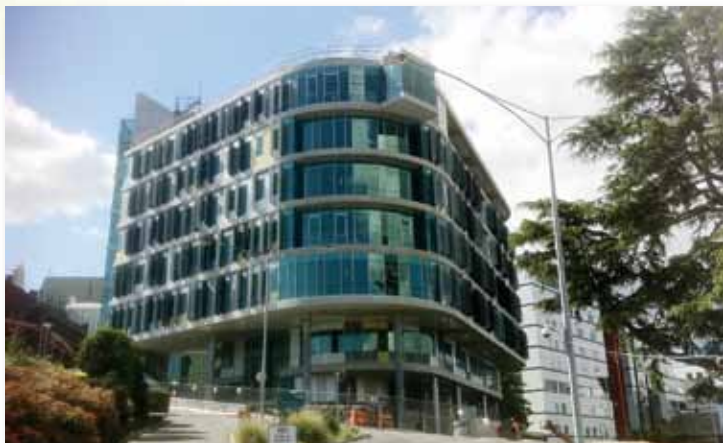
External structure almost finished
