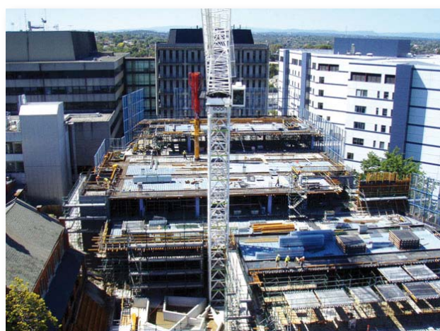
Level 6 North is currently under construction
