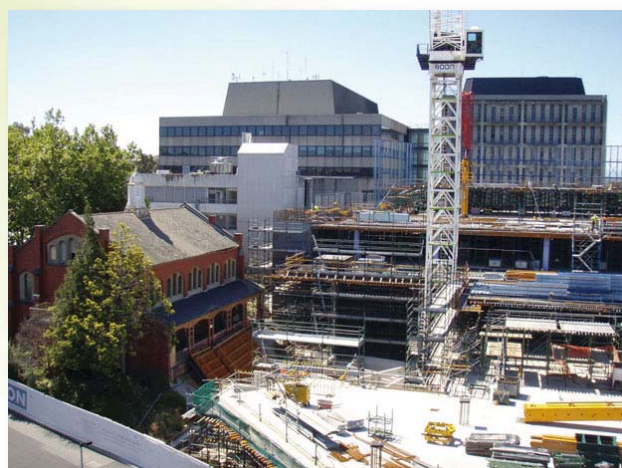
Level 5 North is now complete
