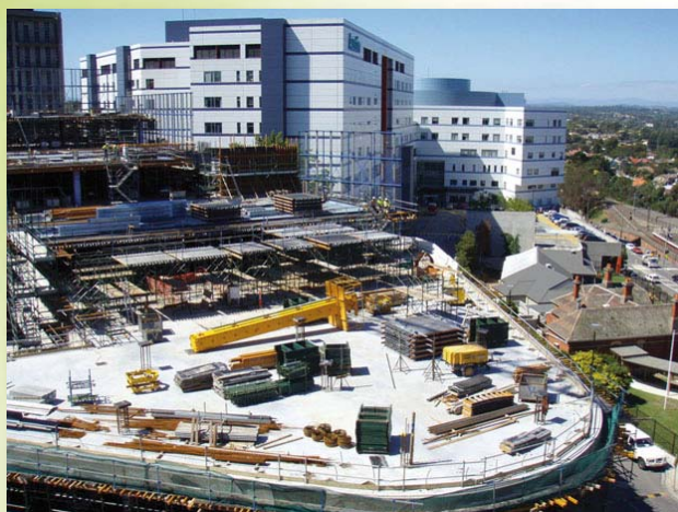
Level 4 South is almost complete
