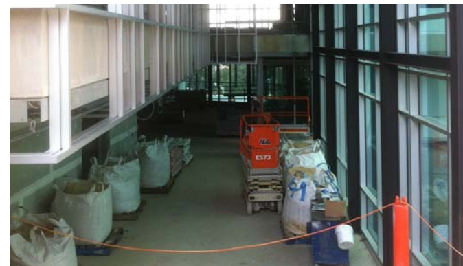
Full steam ahead on internal fitout.
