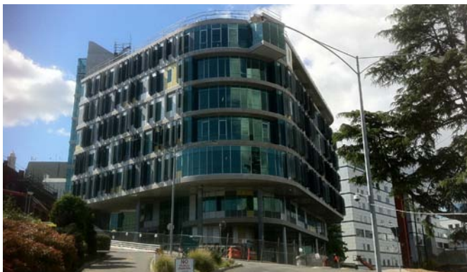
External structure almost finished.
