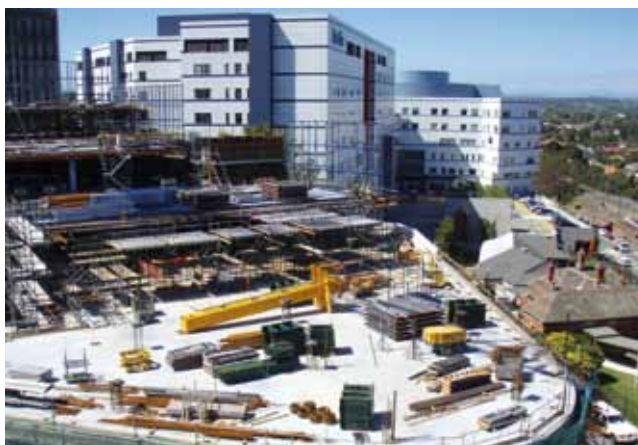
Level 4 South is almost complete.
