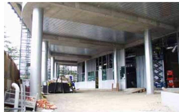
Main drop off area on Level 2 with glazed facade being installed.
